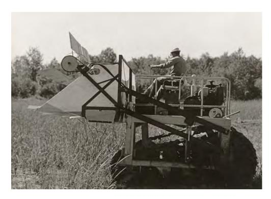
Fig. 1.24 Example of a mechanical harvesting machine for wild rice. *Photograph by Bill Burnson.* 1970.
